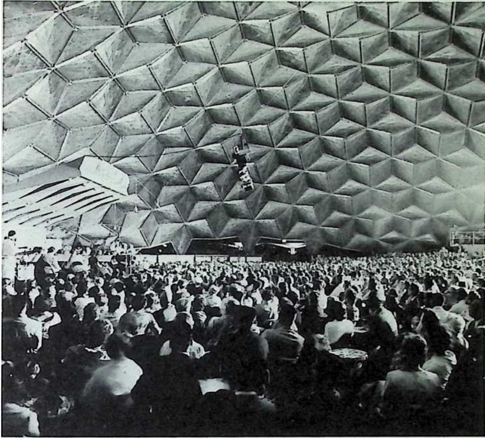
Figure 16.3: Concert audience seated in first Kaiser Dome in Honolulu twenty-three hours after its disassembled components arrived in Hawaii.
