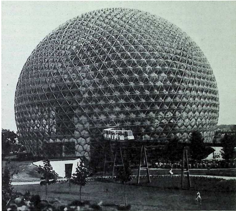
Figure 19.1: Anne's Taj Mahal, the Expo '67 Dome.
