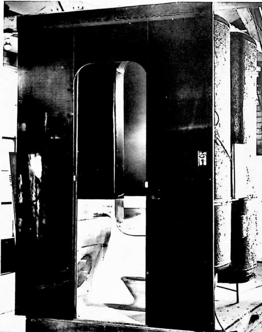
10. Dymaxion bathroom. Complete unit, weight 420 pounds.
