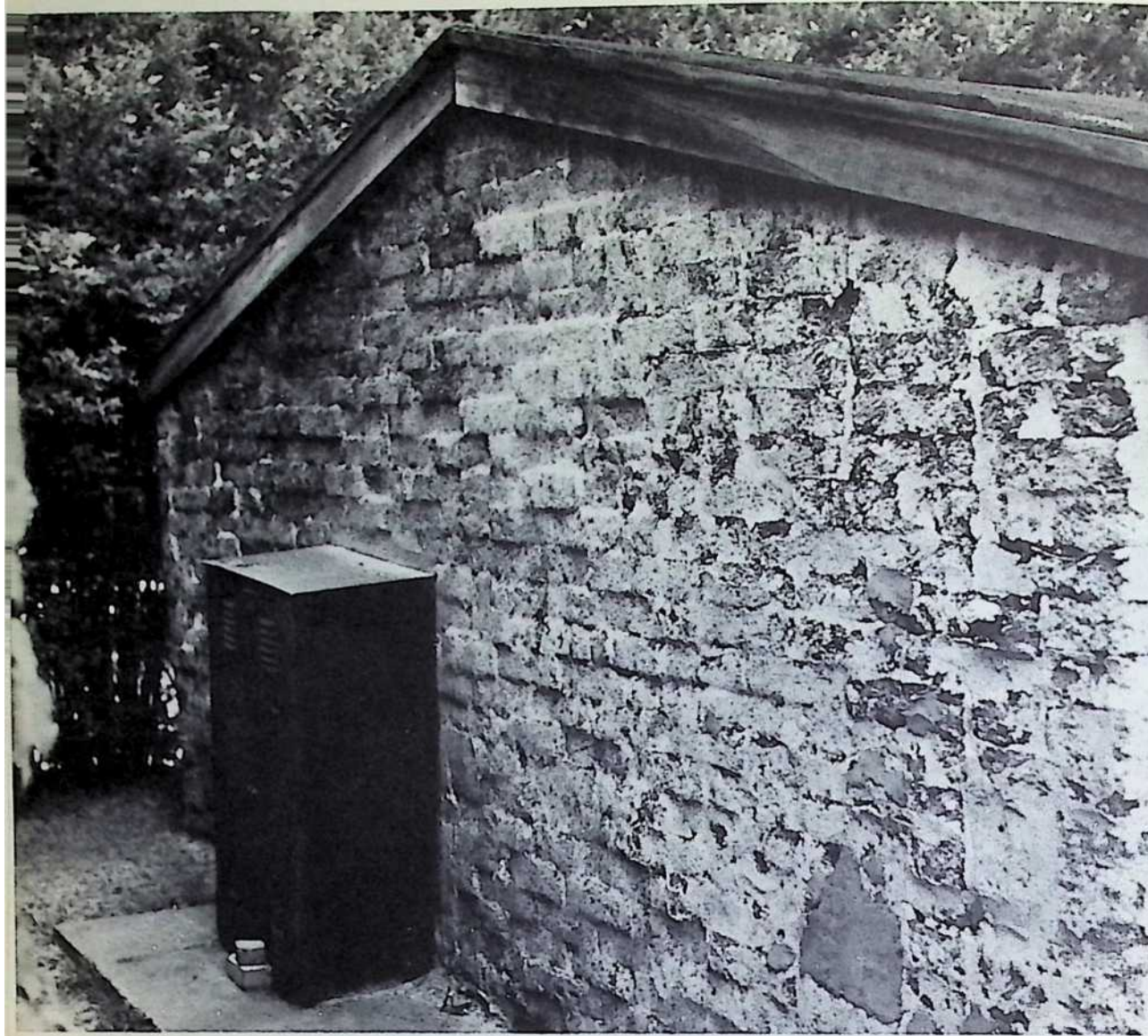
9 A garage wall made of Stockade Blocks still standing in Lawrence, Long Island, on the property originally owned by Fuller's father-in-law, James Monroe Hewlett, co-inventor of the Stockade System and its manufacturing processes. (1923) Stockade walls were a system of reinforced concrete frame construction. The vertical frames were 4-inch columns on 8-inch centers. The cylindrical vertical 4-inch columns were tied together horizontally at every floor height by concrete lintels above and below every door and window opening. This continuous, in-
