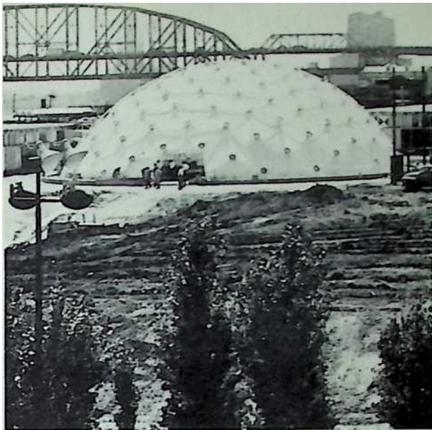
354. Giraffe crane speeded erection of 114-foot Geodesic pavilion at Winthrop Rockefeller's Winrock estate, Hot Springs, Arkansas, 1956.
