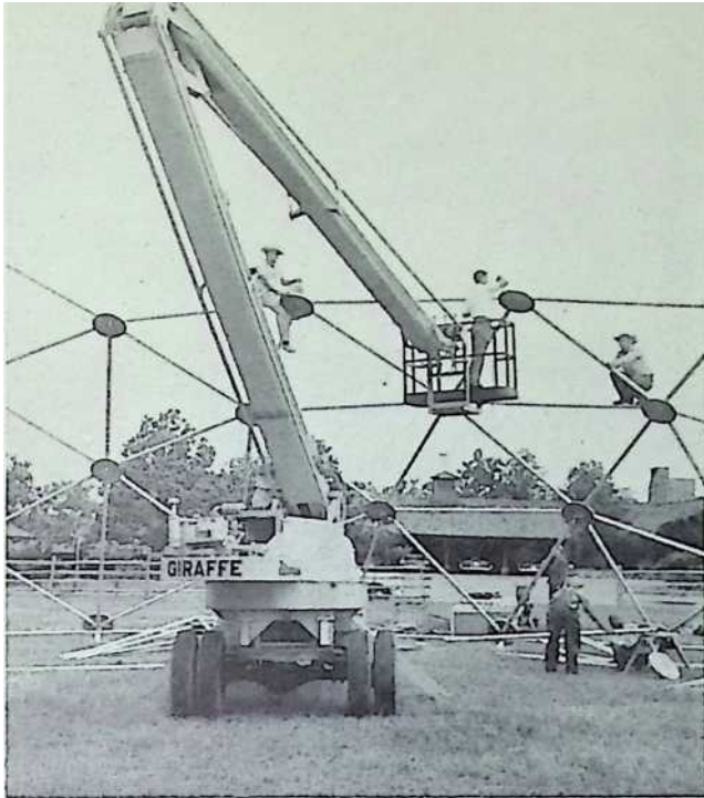
354. Giraffe crane speeded erection of 114-foot Geodesic pavilion at Winthrop Rockefeller's Winrock estate, Hot Springs, Arkansas, 1956.
