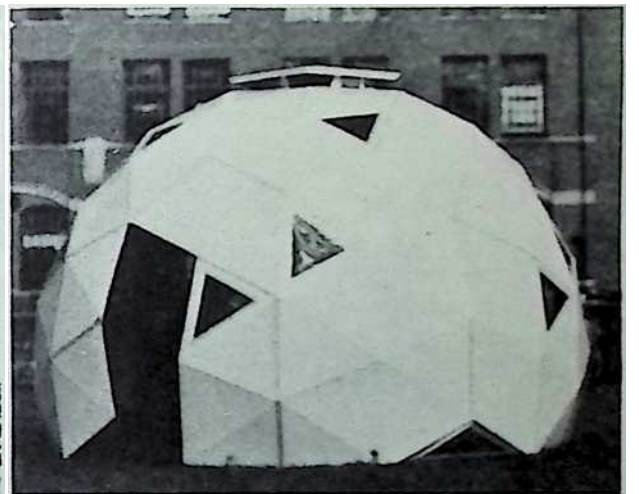
424. Polyester-resin paperboard Geodesic dome, North Carolina State College, 1954-
